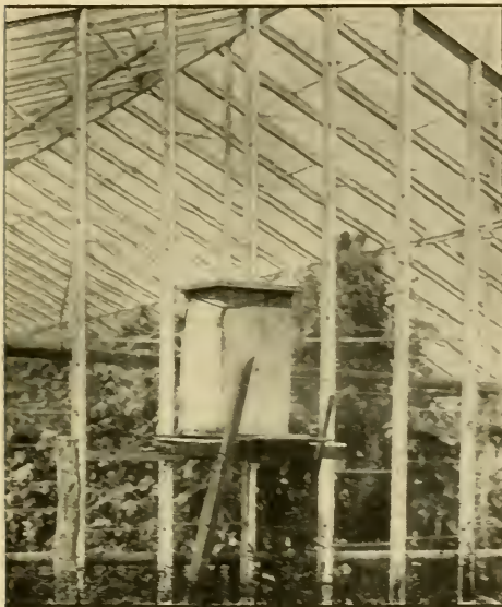
INTERIOR OF CUCUMBER - GREENHOUSE : HIVE WITH ENTRANCE INSIDE.
